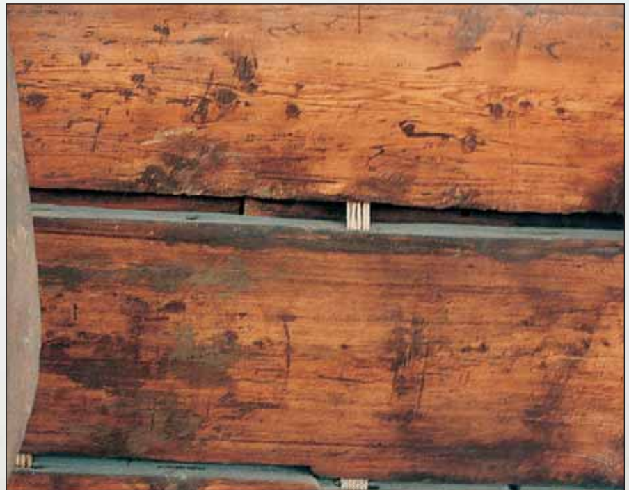
Photo.3: When wet, the ropes would tighten, sealing the well-jointed boards without the need for caulking
